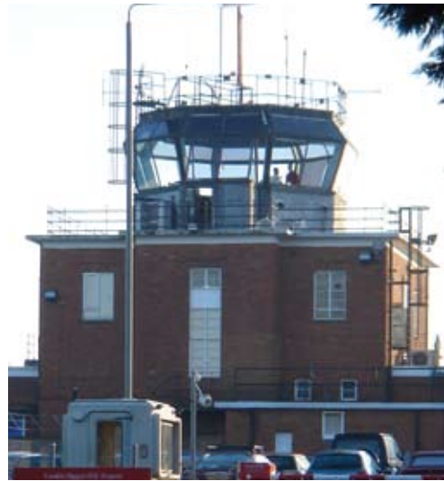
London Biggin Hill Airport control tower
